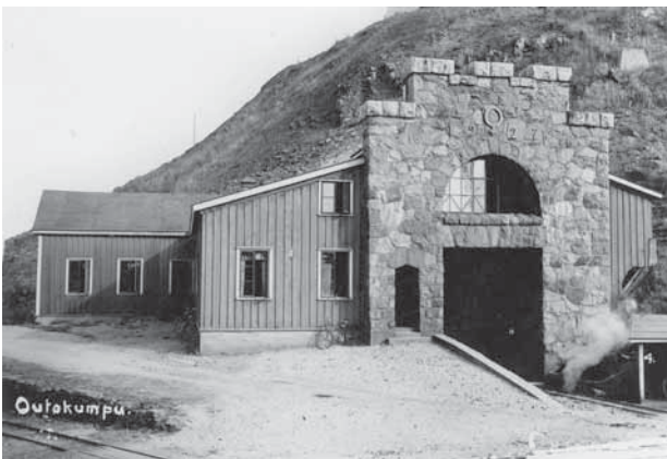
Fig. 6. Washing facilities and changing room for the miners was completed in 1927
