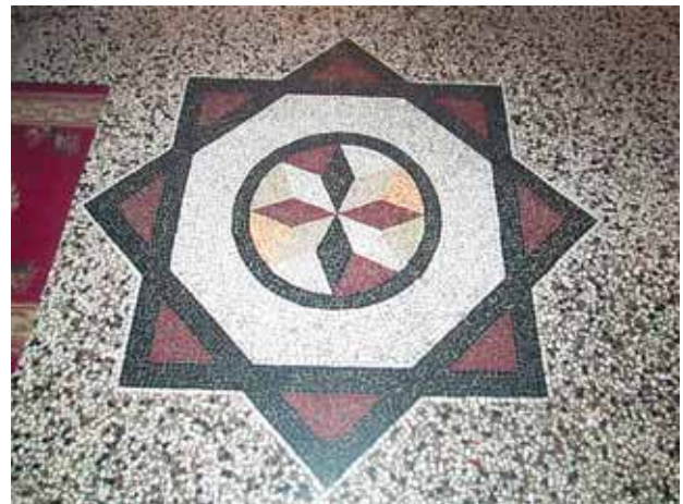
Fig. 4. Element of Flooring in the Church dedicated to the Saint Apostles Peter and Paul
