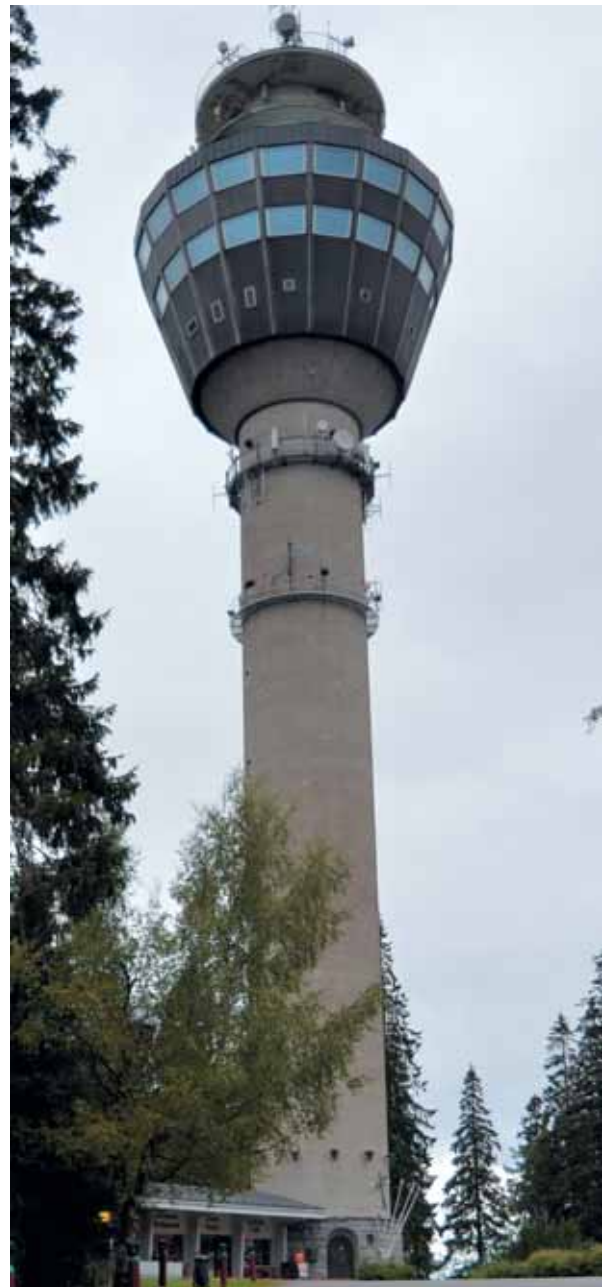
Fig. 7. The Puijo Tower stands 306 meters above sea level and 224 meters above the surrounding Lake Kallavesi. (Photo: Jari Nenonen, GTK)
