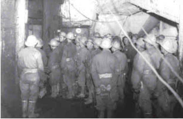
Fig. 5. Miners entering the lift
