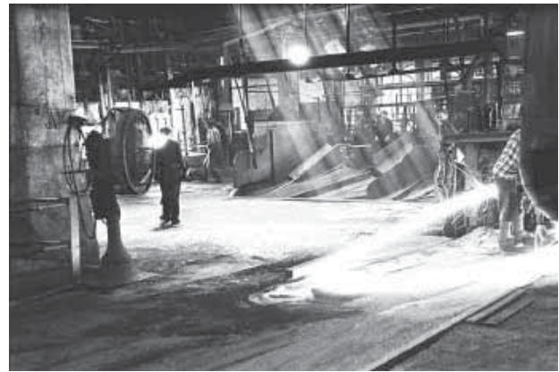
Fig. 13. In the Foundry of Vartsila Plant. The 1970-s
