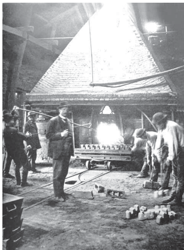
Fig. 7. Ingoting of copper on Pitkaranta plant. G. Grendal, 1896
