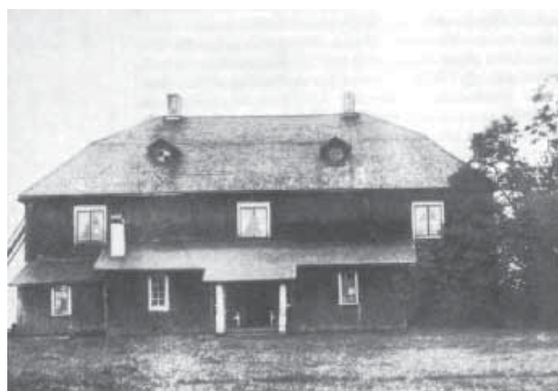
Fig. 3. The house in Palkjarvi (Alahovi).1891
