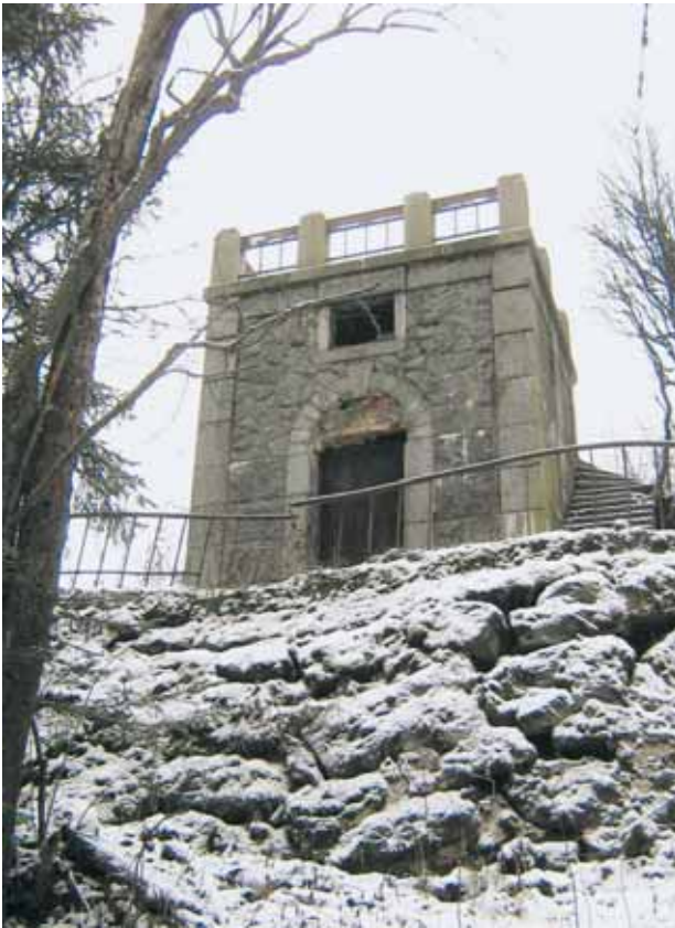
Fig. 2. Water-Tower on Kuhavuori Mountain
