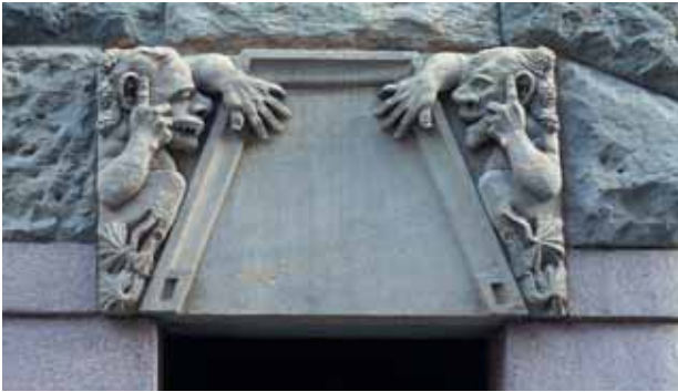
Fig. 29. Soapstone ornamentation incorporated into the facing of a Jugend-style office building in Helsinki, dating from 1901. (Figure: Jari Väätäinen, GTK)
